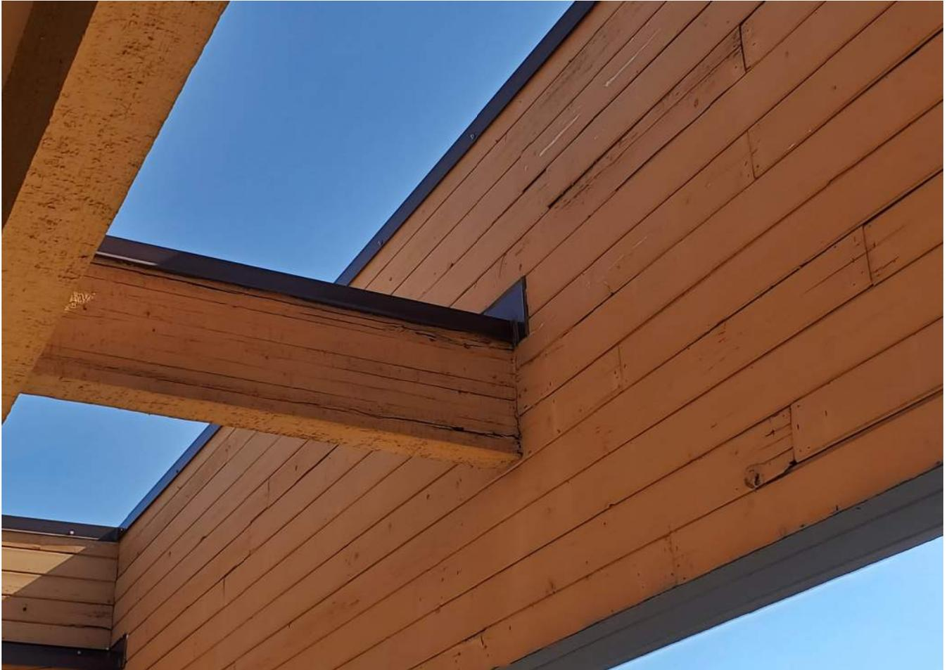
Deteriorated outrigger at east facade
