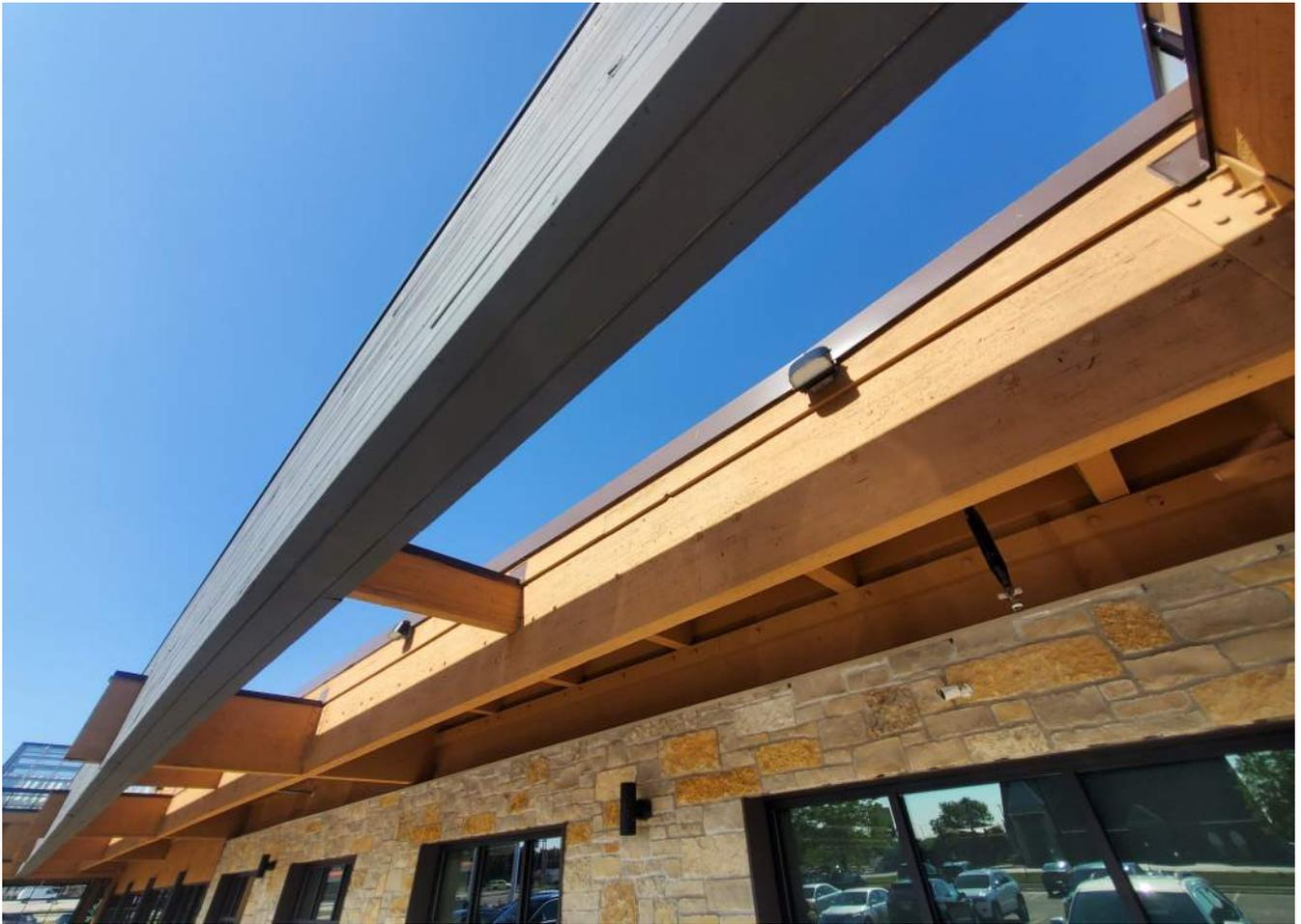
Deteriorated outrigger at east facade
