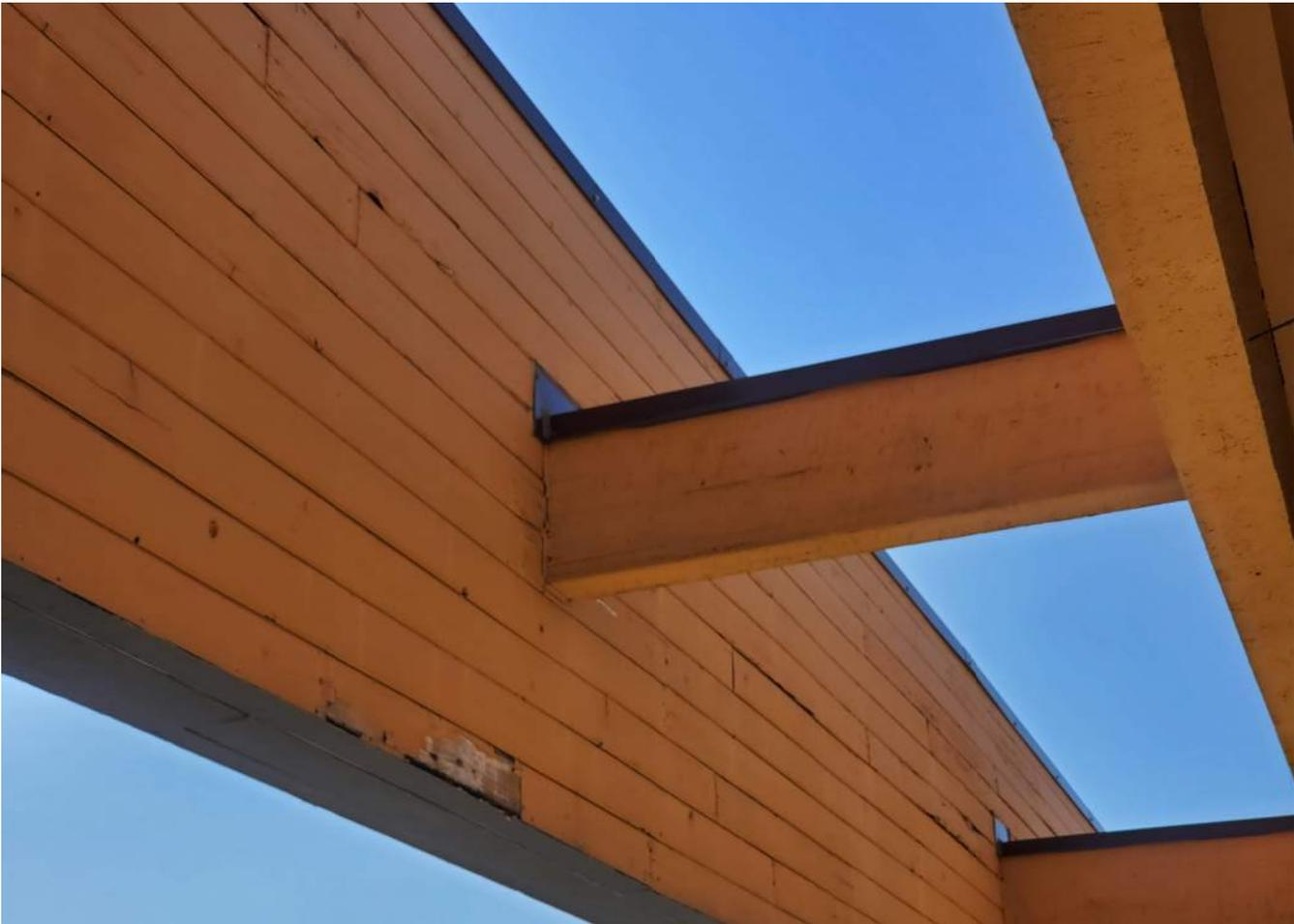
Deteriorated outrigger at east facade
