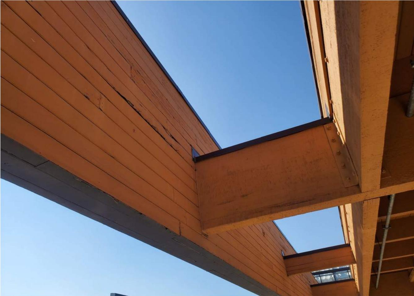
Deteriorated outrigger at east facade
