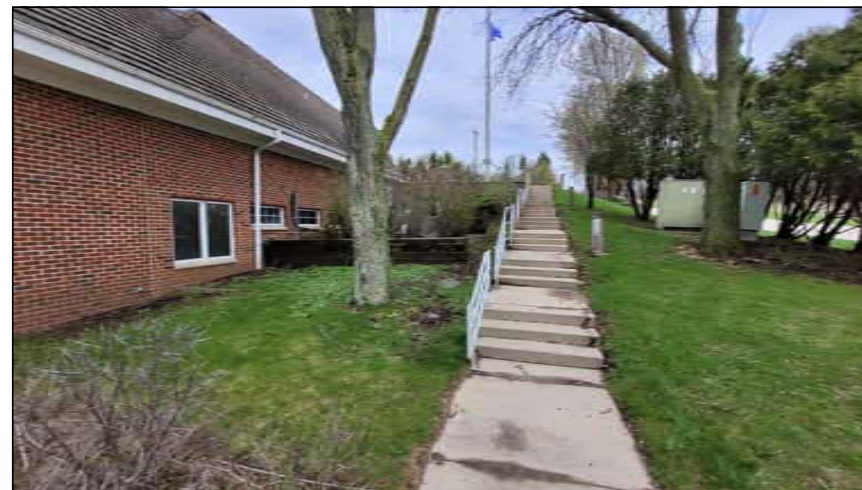
VIEW OF EAST SIDE STAIRS
