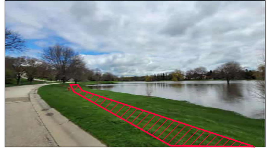
VIEW OF PARK AREA (FLOODED)
