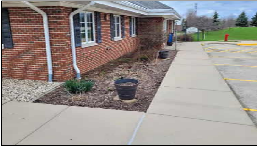
VIEW OF POLICE DEPARTMENT ENTRY
