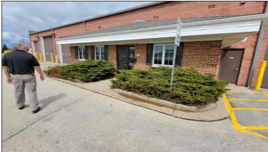
VIEW OF PUBLIC WORKS ENTRY
