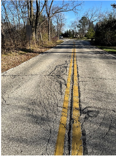
Pavement Deterioration
