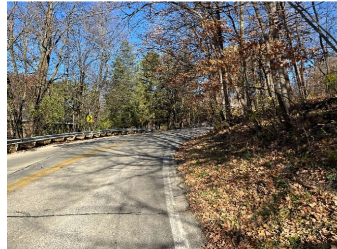
Sight Distance Issues
