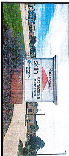
EXISTING - VO IS 116.5" X 21.25", 2" RETAINERS, 2.5" H-BARS
